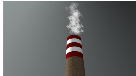
Waste heat recovery
