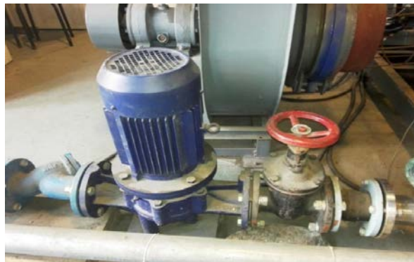
Cooling water pump
