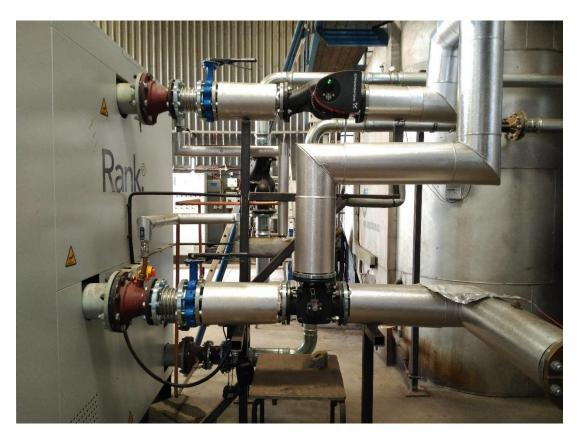
**Combined Heat and Power (CHP)** using **biomass** as renewable heat source
