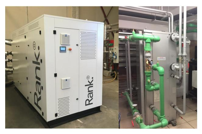
Combined Cold, Heat and Power (CCHP) using solar/biomass as renewable heat source
