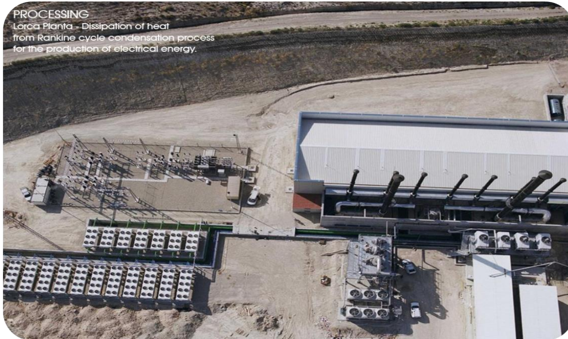
ORC Condenser - Spain
