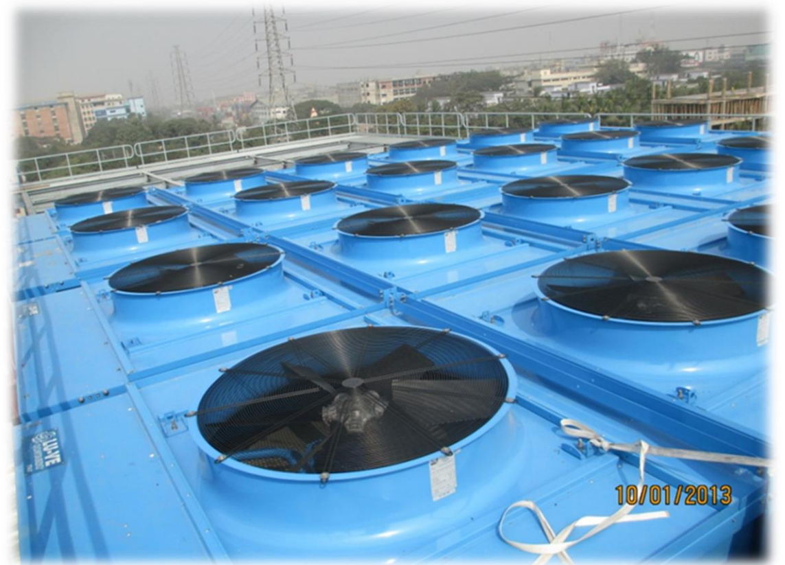
Motor cooling plant - Bangladesh
