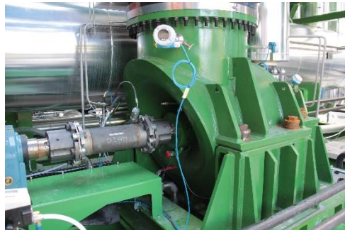
High Temperature Heat Pump Produces high temperature heat from low temperature heat
